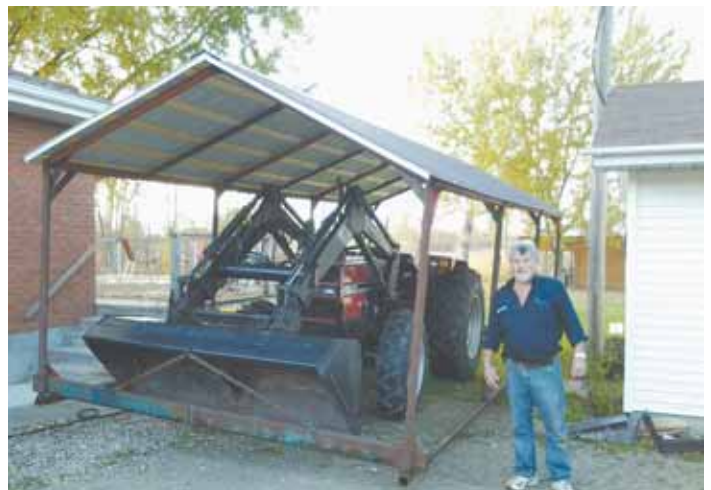
Gary Pierman used 3-in. dia. steel pipe to build this portable storage shed, which he can pick up and move with his Case IH loader tractor.
