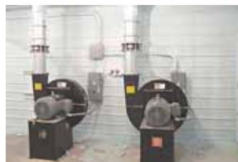
Recirculating system uses 40 hp motors to oxygenate the fish tanks. Air diffusers along bottom of tanks create 2 opposing flows of water.
