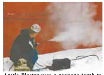
Arctic Blaster uses a propane torch to create dry steam that thaws frozen pipes.
