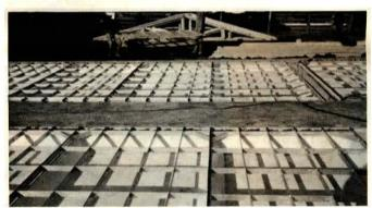
Pans install below grates in new or existing buildings, sealing animals and equipment off from pit gases.
