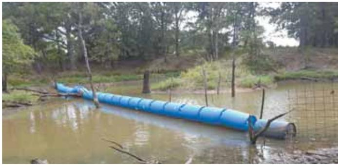
Barrel fence solves the problem of trash catching in wire and other types of fencing. The threaded-together barrels tend to roll right over it.
