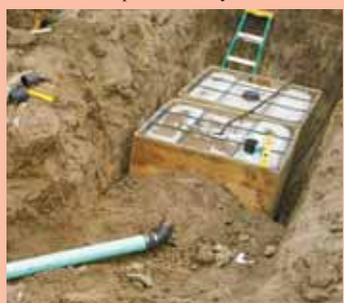
Totes at left being used as a septic tank. Cage, right, employed as hay feeder.
