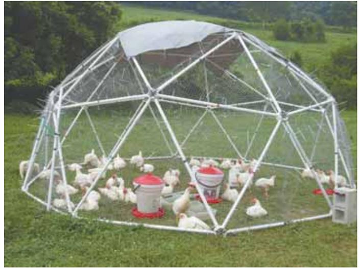
Thanks to the connecting hub design, one person can assemble the frame for a 16-ft. dia. Zip Tie Dome within a couple of hours.
