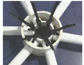
Dome's struts slip into holes on 4-in. dia. pvc hub. Zip ties slip through holes in struts for a secure connection.
