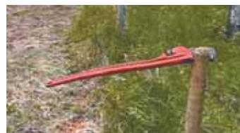
The weight of the clamped-on pipe wrench keeps post from bouncing as Lehmann hammers staples into it.
