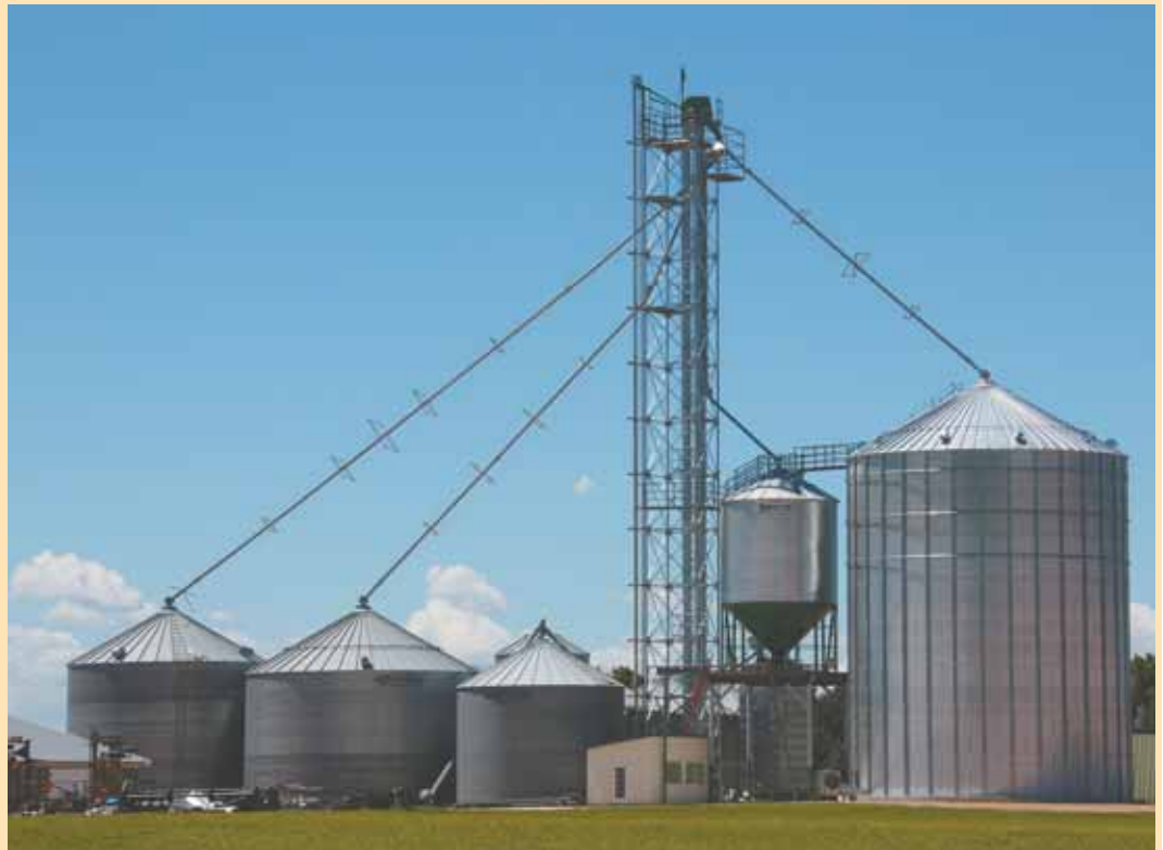
The showpiece of Tim Kelly’s grain handling system is a 120-ft. tall tower. It discharges dry grain through 8-in. dia. spouts to 4 bins, including one with 95,000-bu. capacity.
