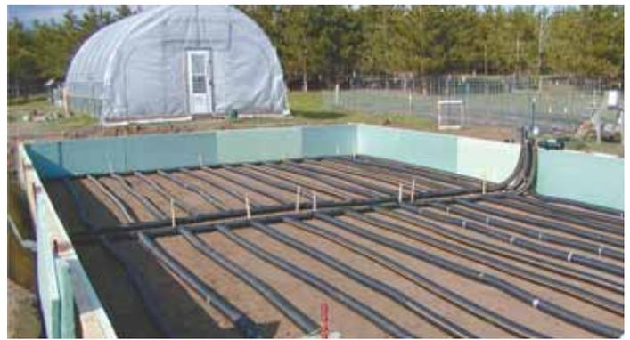
Greenhouse floor is covered with 1 ft. of sand and a series of 4-in. corrugated drain tile on 16-in. centers.
