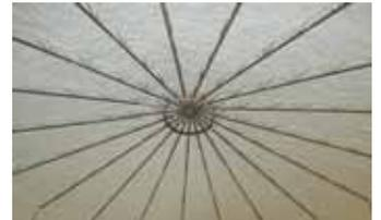
He cut the trusses to the right angle and then cut a 3-ft. long, 9-in. dia. steel pipe to serve as a center collar (above). A telescoping forklift was used to set each truss in place.
