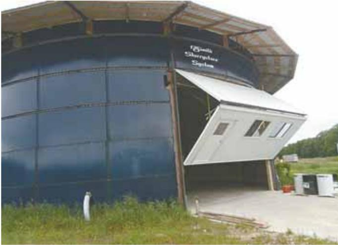
Marv Rubingh converted his 23-ft. tall, 62-ft. dia. Slurrystore into a shop complete with a Schweiss bifold door and barn steel roof.
