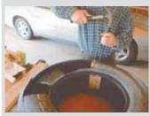
C.F. Marley, Nokomis, Ill.: "You can cut small squares of rubber out of a tire's sidewall by using a wood chisel and a wood block. Just insert a 2 by 4 under the part you want to cut. You can also use a sabre saw by first drilling a hole through the rubber."
