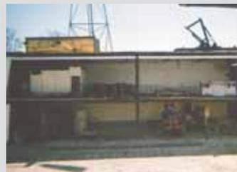
**Reuben Miller, Nappanee, Ind.:** When he bought a load of concrete forms, the old enclosed semi trailer that delivered them came with the deal. They removed one wall and created a shelf inside the remaining shell, mounted on an angle iron frame. The heavy-
