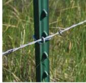
You clip the staple onto one side of post and then use a pliers to bend it around back side of post.
