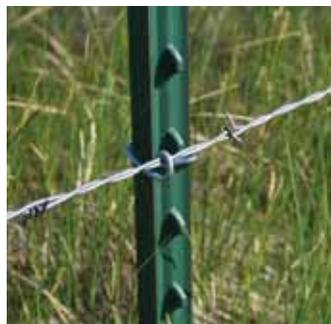
You clip the staple onto one side of post and then use a pliers to bend it around back side of post.
