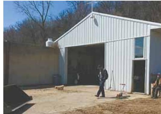
William Benson built this 30 by 60-ft. earth-sheltered shop inside his old concrete trench silo. The silo was dug into a hillside and had slanted-out walls with concrete supports.
