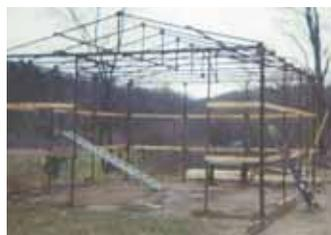
Sonny Barcus welded the building's walls together on the ground and then lifted them into place with a tractor.
