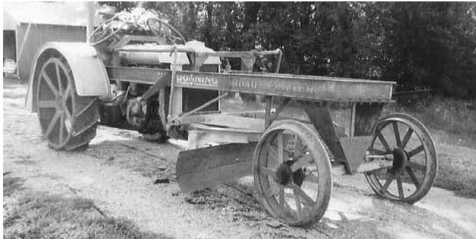
The first powered road grader ever was built by Adolph Ronning in 1924. Arnold Zempel found it disassembled in Ronning's daughter's shed and put it back together.
