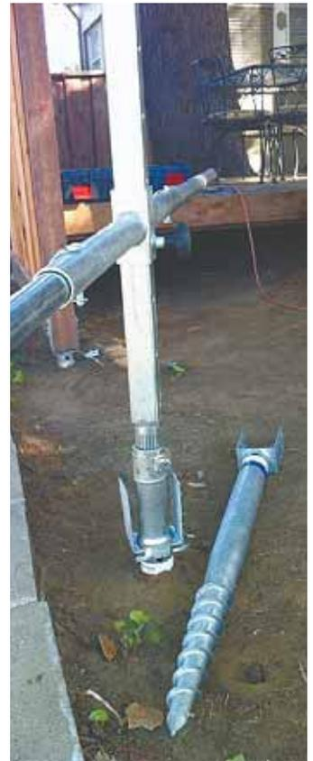
Galvanized steel tube screws into the ground. Post bolts onto a steel plate welded to top of tube.
