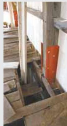
Spliced sections were reinforced with channel iron and steel plate.
