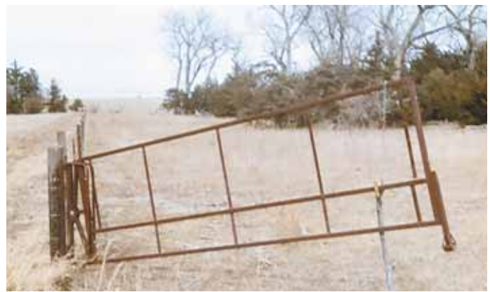
Gate pivots up or down over uneven terrain without binding.
