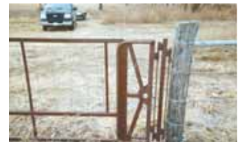
Pivot hinge attaches directly to gate post. A second hinge can be mounted on end of gate to attach to a second section of gate to make an extra-wide, flexible gate.
