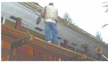
When Alan Shelbourn added a second floor to his house, he built catwalks to make it easy to clean out gutters. The walkways connect to a large deck at one end of his house and the garage at the other.
