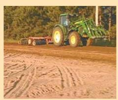
Farm equipment is all that is needed to prepare the soil and mix the solution. An industrial roller or packer will do the best job compacting. Discs and rototillers may also be used to mix the soil. After the correct grade is achieved, compacting is key.
