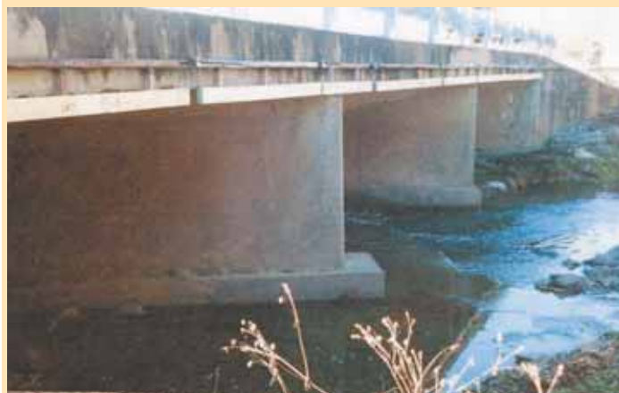
Phillip Poston took advantage of reinforcing steel bars on the downstream side of this bridge to build a "breakaway" fence across the creek that runs through his pasture.
