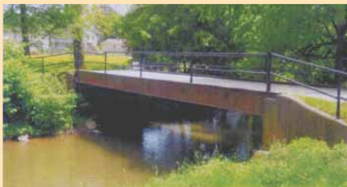
Sam Stoltzfus and his cousins built this 14-ft. wide by 48-ft. long bridge across a creek, allowing access to a township road with little traffic.
