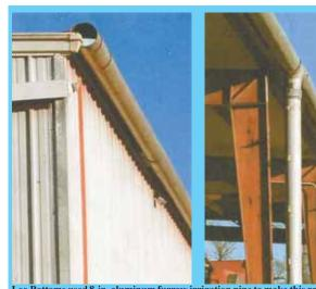
Leo Bottoms used 8-in. aluminum furrow irrigation pipe to make this rain gutter system for his 75 by 150-ft. shed. The gutter downspout empties into an underground pipe that runs to a nearby pond.
