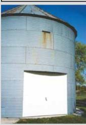
Howard & Gary Reischauer, Zearing, Iowa: To make a storage building for smaller equipment and tools, the Reischauer's cut an opening into a 3,000-bu. grain bin by framing it with 2 by 5 studs and a header. They installed a single manually-operated garage door in the opening.
