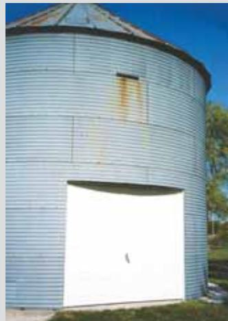
**Howard & Gary Reischauer, Zearing, Iowa:** To make a storage building for smaller equipment and tools, the Reischauer’s cut an opening into a 3,000-bu. grain bin by framing it with 2 by 5 studs and a header. They installed a single manually-operated garage door in the opening.
