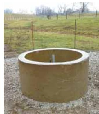
The 4-ft. dia. concrete culvert has a floor made of Quikcrete and is fed by an artesian well.
