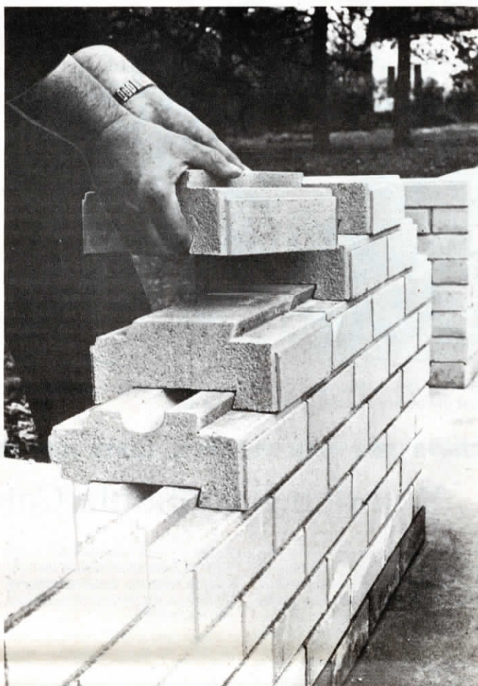
New Zip bricks interlock, allowing you to construct straight, sturdy walls without mortar. You can use them to divide a room or basement, build a fireplace, or a decorative fence and many other uses.
