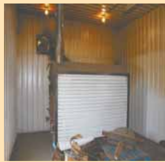
The Hall family burns corn cobs to heat their 12,000 sq. ft. shop (left) and their 1,500 sq. ft. temporary living quarters. A separate building 50 ft. from the shop (above right) houses the cob burner and cob storage (above and at right). An elevator at back corner of cob storage unit loads cobs into stove.
