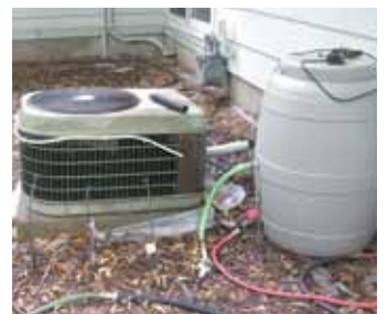
Do-it-yourself mister keeps air conditioner's fins wet so it cools better.
