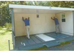
Once the shelters are in place, the 26-ga. steel-sided walls can be easily erected by 2 or 3 people in just a few minutes.
