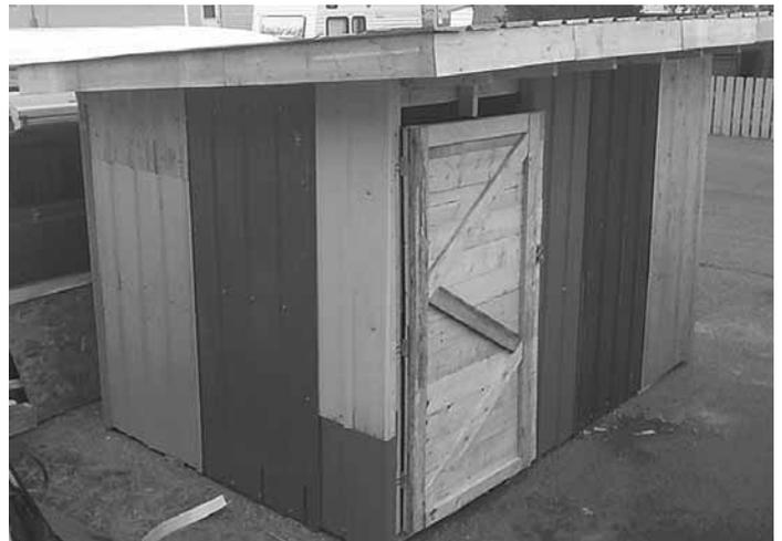
He made the shed 2 pallets wide by 3 pallets long, with 2 by 4's around the perimeter and lengthwise down the center.
