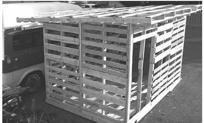
Dave Mathia built an 8 by 12-ft. shed (shown here under construction) mostly out of pallets and other recycled materials. His total cost was less than \$100.
