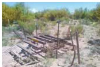
David Shumway used 8-ft. wide steel joists out of an old semi trailer to build this ATV cattle guard.
