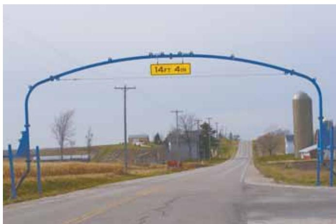
Chad Tasch uses a telehandler to set up his 20-piece “pipeline bridge” for liquid manure. Its end supports rest in roadside ditches, out of the way of passing traffic.
