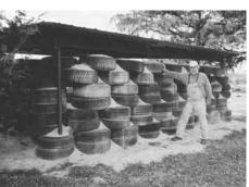
He stood in a loader bucket and used a sledge hammer to drive the steel posts into the ground, without using any concrete as anchors. To help keep the roof from sagging, in some places he welded horizontal steel plates onto the posts. "The plates are wedged in between the tires so the posts won't sink into the ground," notes Myrick.
