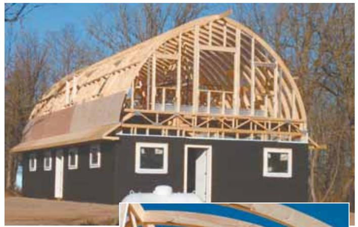
Del Stubbs loves the clear span, open space design provided by the Gothic arch roof on his two-story, 26 by 50-ft. workshop. He nailed tapered 2 by 4's together into a rib-like assembly to create the peak's pitch.
