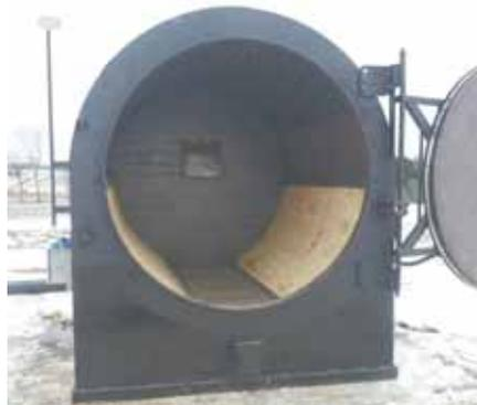
Willie Albrecht uses this stove to burn soybean bales. Hot water is piped into his shop's in-floor heating system.
