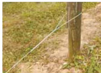
Dead ends (left) create a secure loop around a post or a 90 degree turn around a corner post. Splices are said to be stronger than original wire's breaking strength.
