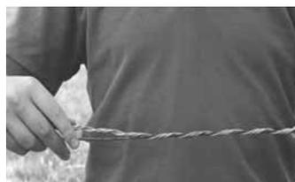
Wrapping the splice around a broken wire, or the dead end to a terminating wire at an end post, creates a solid, rod-like connection.
