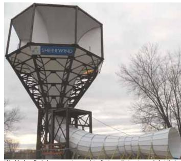
"Upside down" wind energy system consists of a tower that captures wind at the top and funnels it down through a tapering passage, which accelerates the flow and feeds into turbines to produce power.
