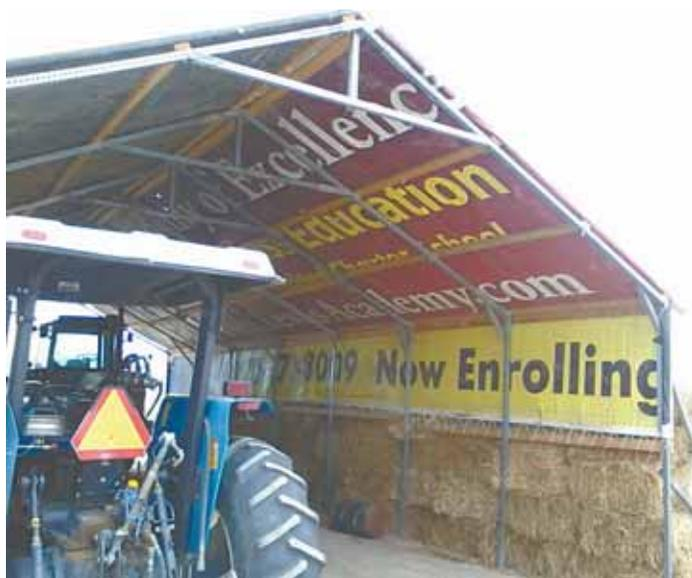
To make this machine shed, Ted Carlson sewed two 40-ft. plastic billboard tarps together and then stretched them over wooden trusses to make a watertight roof.
