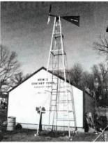
We used a truck engine fan to make blades for the windmill, extending the blades so total blade diameter is 48-in. We used a Ford car spindle for the hub. We used a car wheel balancer to balance the blades. The windmill is 6 ft. square at the base and its legs are anchored in 5-ft. deep, 12-in. dia. cement pillars. We also built a second 10-ft. tall windmill.
