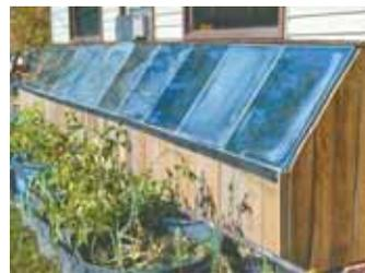
Hot air is pulled from solar heater and fed into the house by a blower. Before the hot air is dispersed, it passes through a furnace filter to keep out dust and debris.
