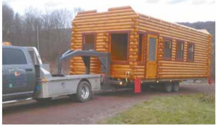
Log cabins are fully assembled in widths up to 12 ft. wide and lengths up to 32 ft. long before delivery. The roof section is added onsite.
