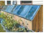
Hot air is pulled from solar heater and fed into the house by a blower. Before the hot air is dispersed, it passes through a furnace filter to keep out dust and debris.
