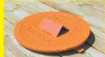
I belong to a rural water district, and to read my water usage I always had to lift the lid off the water meter box. To make the task easier I mounted a handle on the lid by welding a 6-in. length of 1 1/2-in.
