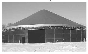
Project manager Paul Hofer reduced the slurry tank's 23-ft. high walls to 18 ft. and cut out holes for an entrance door and overhead door.
