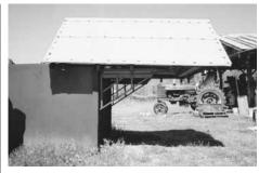
Rolling roof on well house allows James Padgett to pull up a bad well without having to tear the roof off.
