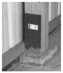
To put up sidewalls, fill posthole with concrete and set professionally-engineered Pier System bracket into it.
