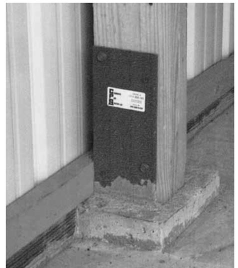
**To put up sidewalls, fill posthole with concrete and set professionally-engineered Pier System bracket into it.**
