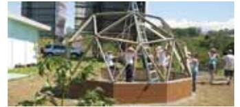
Domes are constructed with 2 by 4-in. wood struts. This model is 15 ft. in dia. and 9 1/2 ft. high.
