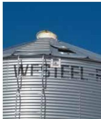
James Haskins installed a sight gauge on his grain bin to prevent overfilling. It extends into the bin 1 3/4 in. with a 1 3/4-in. hole in the middle.
