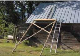
Ladder stands on narrow platform at top of 7-ft. wide wooden brace.
